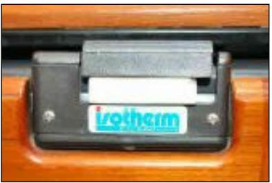
appears to be a simple remedy to enhance the security. It was to stuff a rubber from the chart locker in the catch, which just happened to be of the correct size to force the catch up further and improve its security. This is shown in place in the photo, where the rubber is in place.
